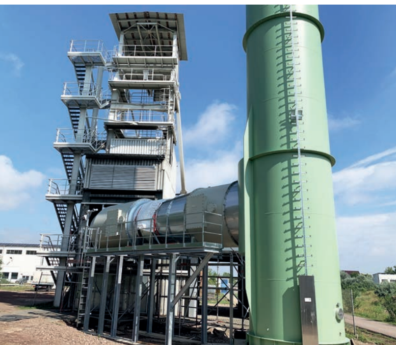
Teutschenthal backfill mine in Germany
