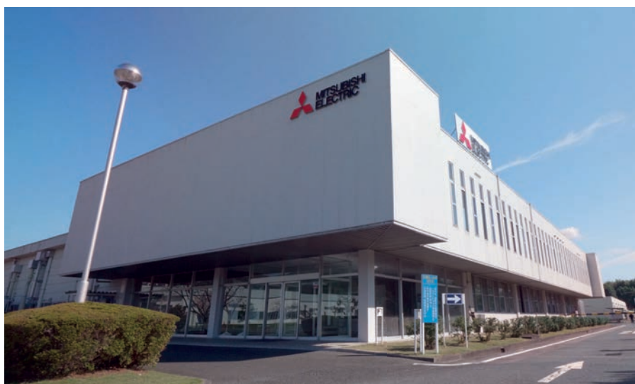
Mitsubishi Electric's Nagoya Works Shinshiro Factory has manufactured three-phase motors since its establishment in 1974.
