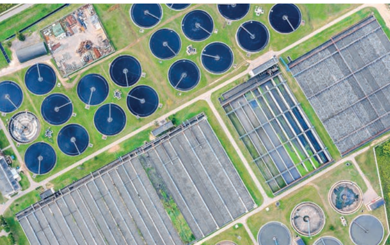
Aerial view of the wastewater treatment plant
