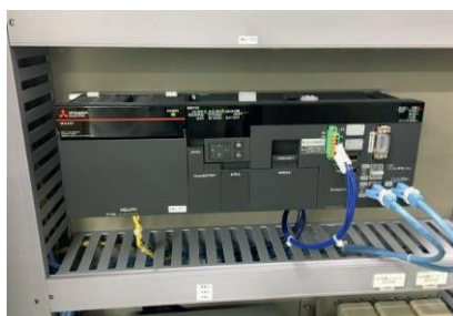
The Real-time Data Analyzer (left) is running in the Mitsubishi Electric "MELIPC" industrial PC where it gathers and analyzes data and conducts diagnostics
